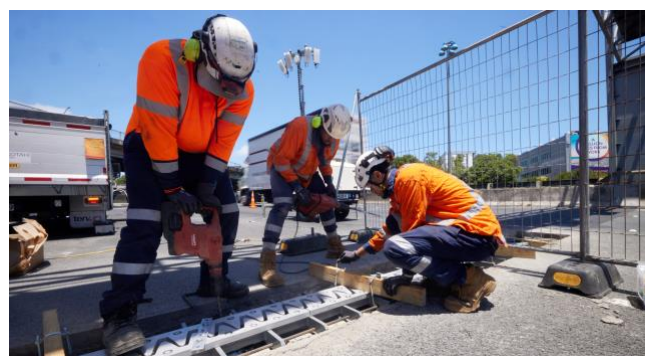
Image 4 Crew installing the new joint with two lanes operating during the day with two lanes of live traffic.
