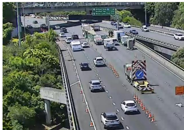
Image 2 Lane configuration of Grafton Bridge No 2 during joint replacement. Image shows two lanes of live traffic with full width lanes.
